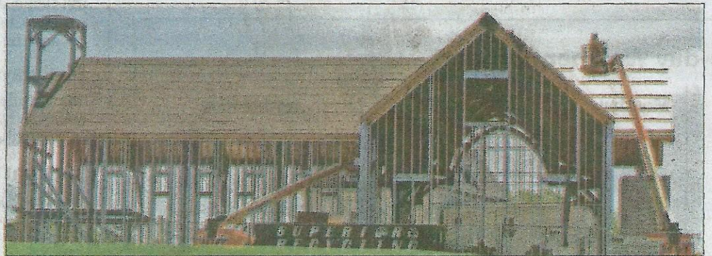
A worker in a lift is framed by the newly installed steel wall supports and the wooden roof structural beams as construction continues on the rebuilding of St. Michael the Archangel Church, on Liberty Street in Pawcatuck, on Friday.
