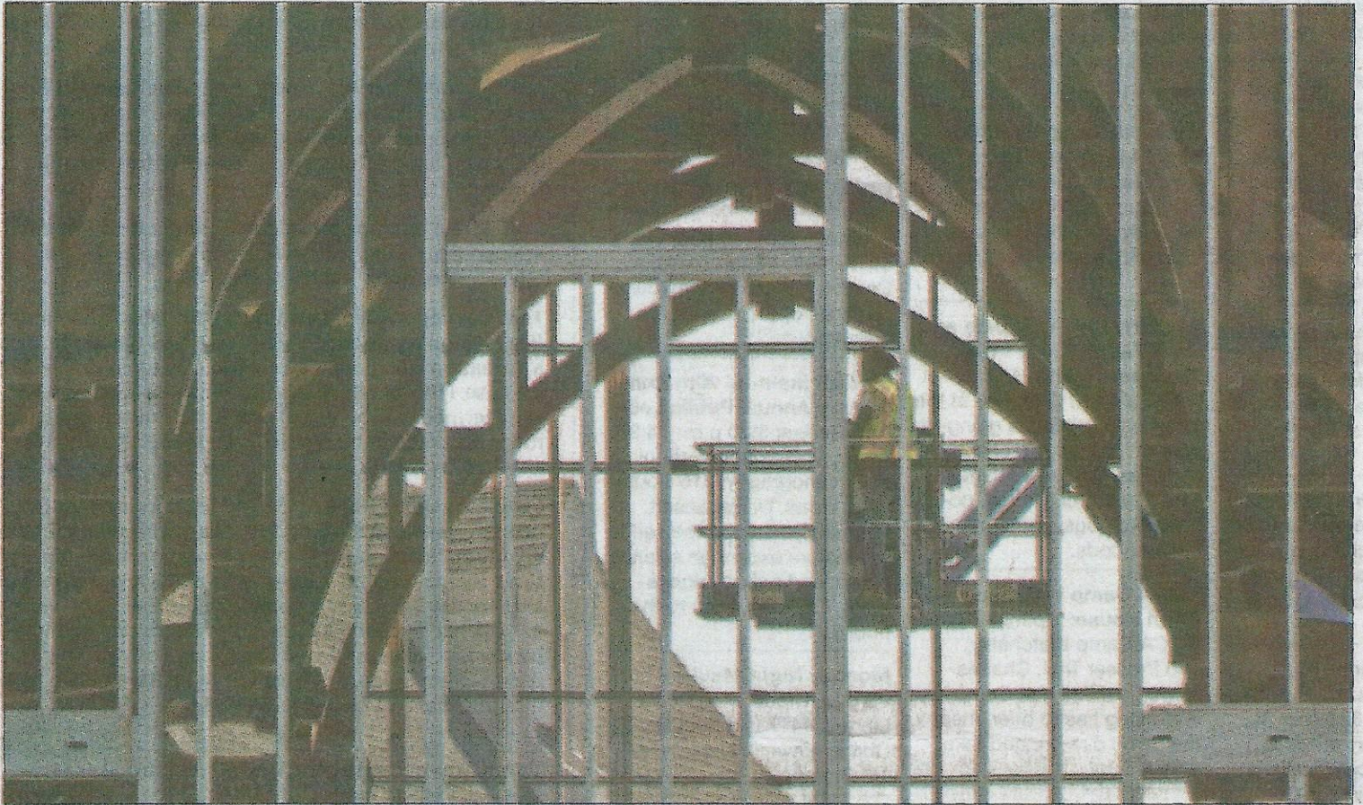
A worker in a lift is framed by the newly installed steel wall supports and the wooden roof structural beams as construction continues on the rebuilding of St. Michael the Archangel Church, on Liberty Street in Pawcatuck, on Friday.
