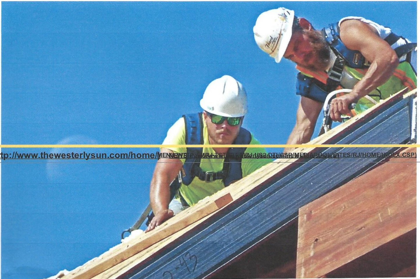
With a waning gibbous moon above, workers with Foard Panel Inc., out of West Chesterfield, N.H., continue the process of installing large pre-fabricated roof panels atop the steel framework of the new St. Michael Church in Pawcatuck on Thursday, May 18, 2017. | Harold Hanka, The Westerly Sun
