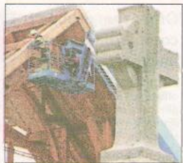
Workers from Foard Panel Inc., based in West Chesterfield, N.H., began installing large, pre-fabricated roof panels atop the steel framework of the new St. Michael the Archangel Church in Pawcatuck on Friday.
