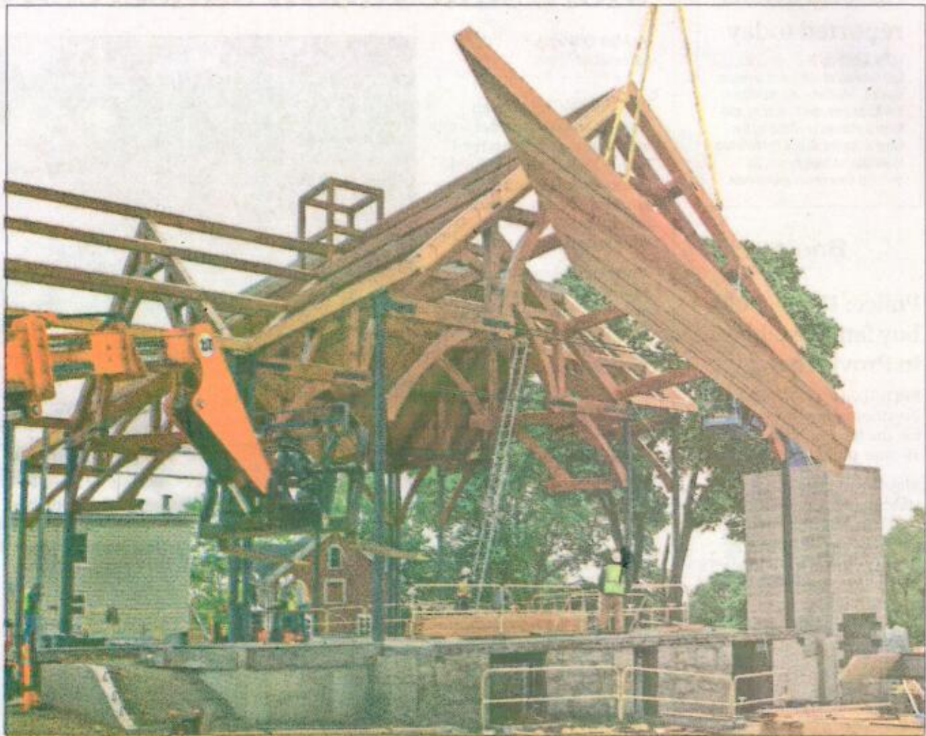
Workers from Foard Panel Inc., based in West Chesterfield, N.H., began installing large, pre-fabricated roof panels atop the steel framework of the new St. Michael the Archangel Church in Pawcatuck on Friday.
