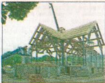
Workers from Foard Panel Inc., based in West Chesterfield, N.H., began installing large, pre-fabricated roof panels atop the steel framework of the new St. Michael the Archangel Church in Pawcatuck on Friday.
