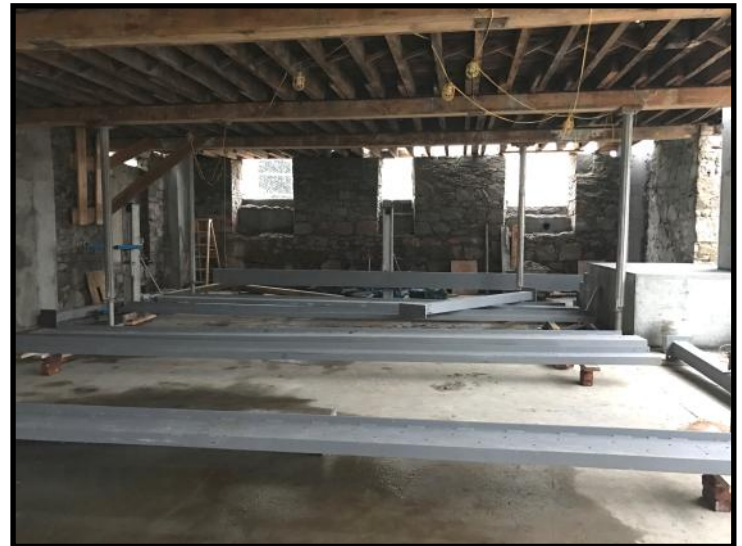
Steel c-channel beams being prepared for installation in the hall area.
